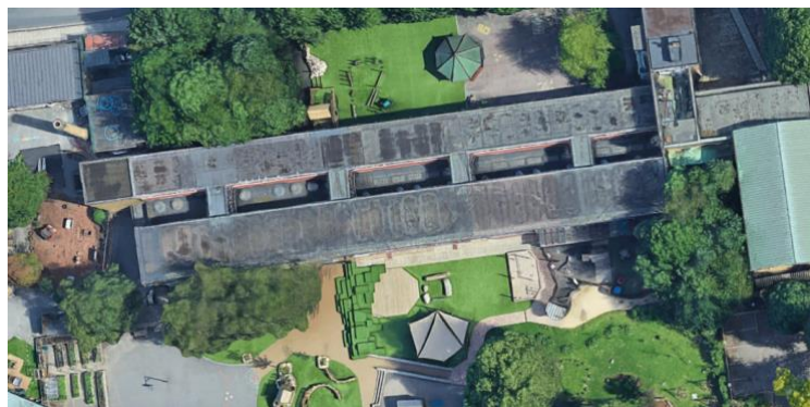
Aerial photograph of Lansbury Lawrence School
